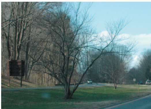
On the George Washington Memorial Parkway, support structures and poles are finished with a brown color to reduce contrast. When all supports and sign backs are treated this way, the roadway character is transformed.
