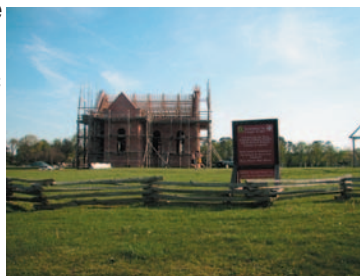
Chapel reconstruction, St. Mary's City
