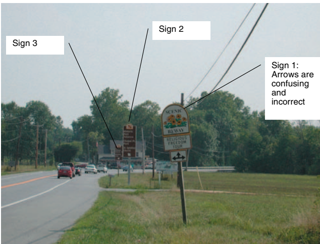
Existing directional signs approaching Port Tobacco on MD 6
